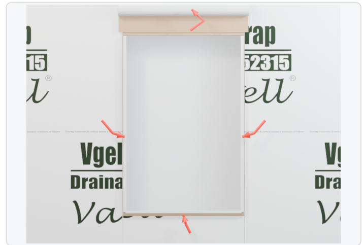
FIG 2 Fold the tabs into the opening.
