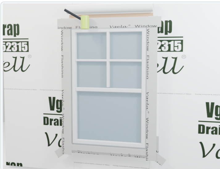
FIG 9 Lap the head strip over the jamb strips.
