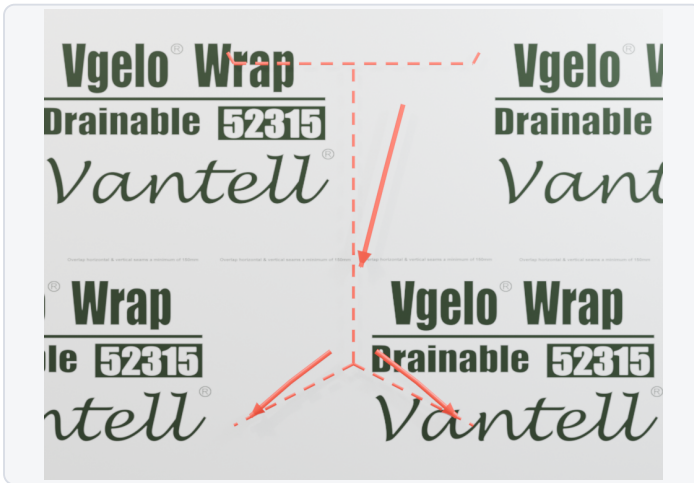
FIG 1 Cut the opening pattern.
