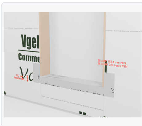
FIG 5 Install the first sill-flashing layer.
