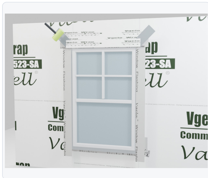
FIG 16 Tape both upper corners with VWFAXW and pressure-roll.
