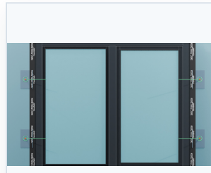
Figure 10. Outboard frame and fixing brackets installed.
